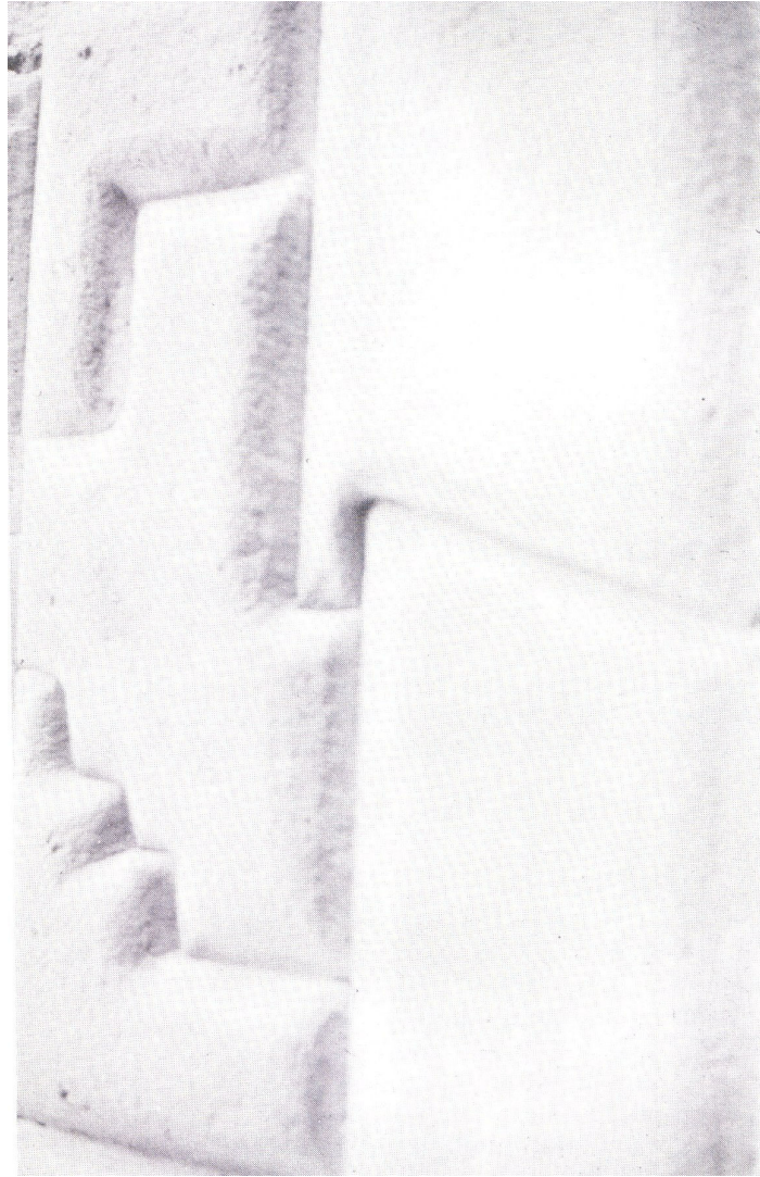
Fig. 17-3. Wall stone with fourteen visible sides, each of which interlocks exactly with adjoining stones. Cuzco, Peru.
